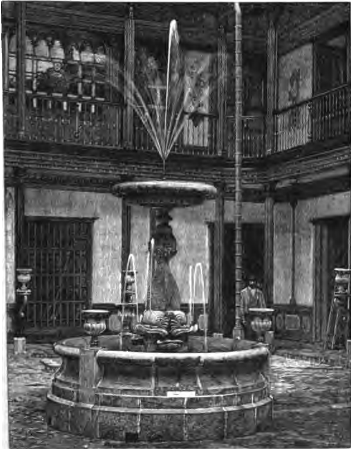
INTERIOR COURT OF A CARACAS HOUSE.
